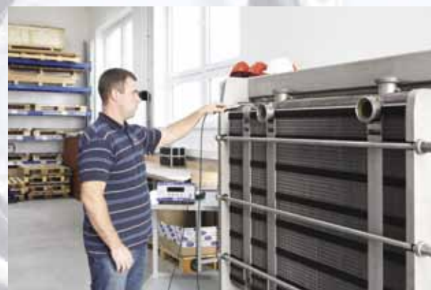
Inspection of plate exchanger packing
